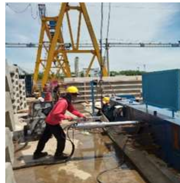
Gambar 9. Proses Stressing
