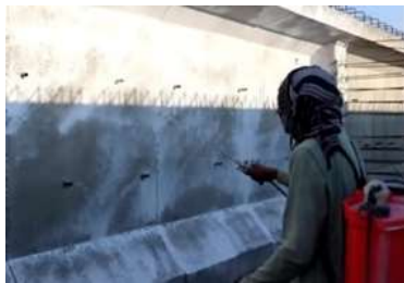
Gambar 15. Curing Compound
